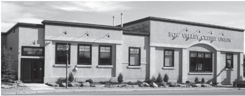
Existing branch at 1st Avenue NE and Main Street, Airdrie.
